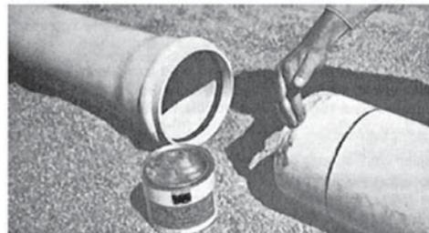
**Step 4:** Insert and push lubricated spigot past the gasket into the bell until the guide mark on the spigot is meets the end of the bell. It is usually possible to manually insert the spigot into the bell on pipe sizes 3" and smaller. Mechanical assistance may be needed for insertion on larger sizes. The "bar and block method" can be used, which allows the installer to feel the amount of force being used and whether the joint goes together smoothly.
