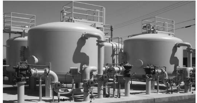
MetalEase-61 Installation in Elk Grove, California
